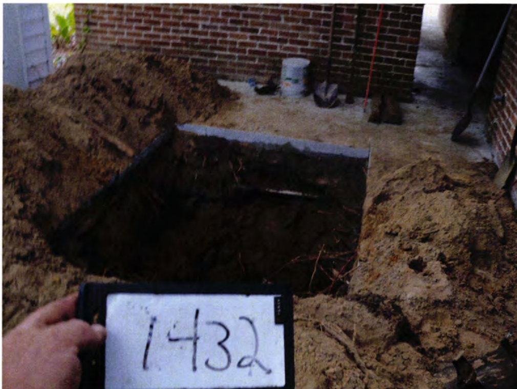
Picture 2: UST 1432Dove excavation pit.
